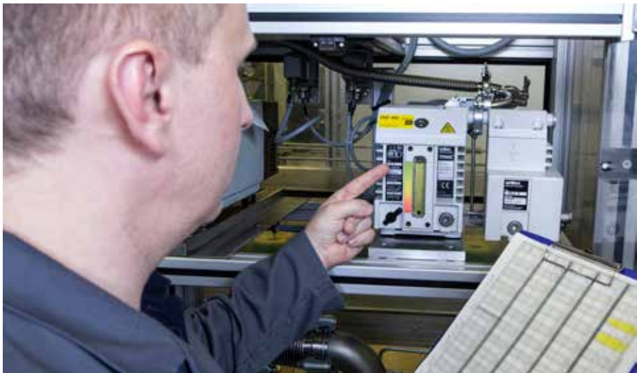
Figure 25: Check before restart; oil level in compliance with specification?
