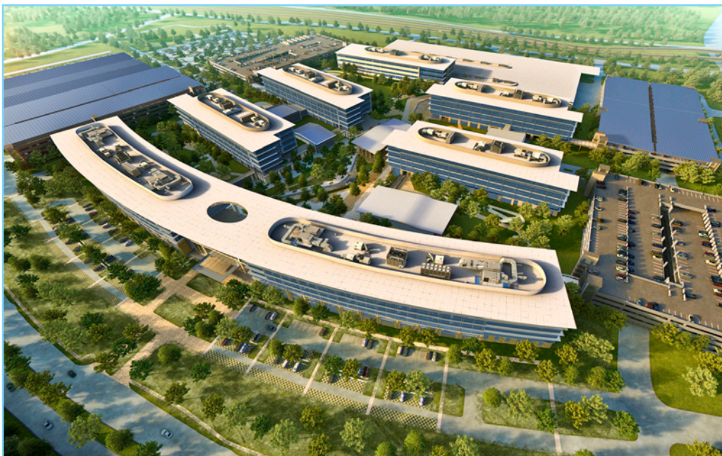
Toyota's new North American headquarters campus in Plano, Texas, will be powered by a 7.75 megawatt solar array that will provide an estimated 25 percent of the campus' energy needs. The system will be the largest on-site corporate office solar installation among non-utility companies in the state of Texas. Completion of the Plano campus is expected in early 2017.
