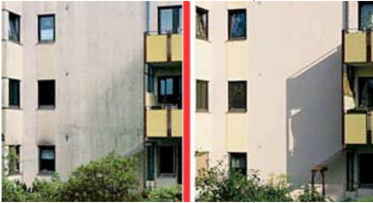
This dirt resistant paint manufactured by Lotusan was designed after the natural self-cleaning mechanism of the lotus flower. www.lotusan.de/lotusan/_o4_faq/index.jsp
